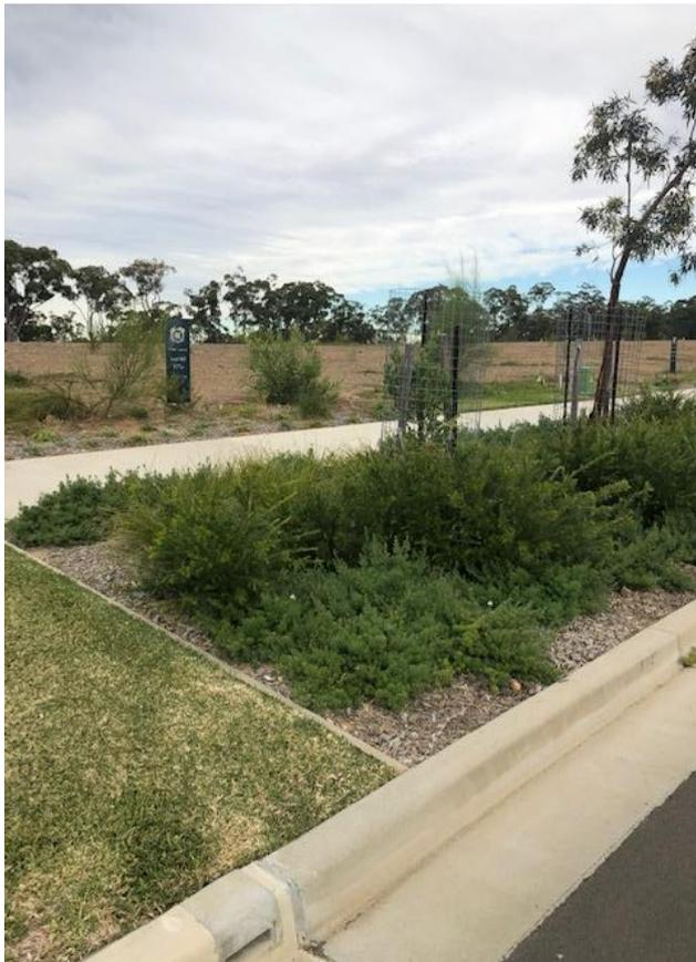
The road-side nature strips or verges are maximised in width, being 3 metres of turf and biodiversity gardens allowing for the planting of large canopy trees, or the retention of existing trees, up to the footpath, and another 1m width of absorbing turf before the property boundary. *The Glenlee proposal has very narrow verges of less than 2m widths.*
