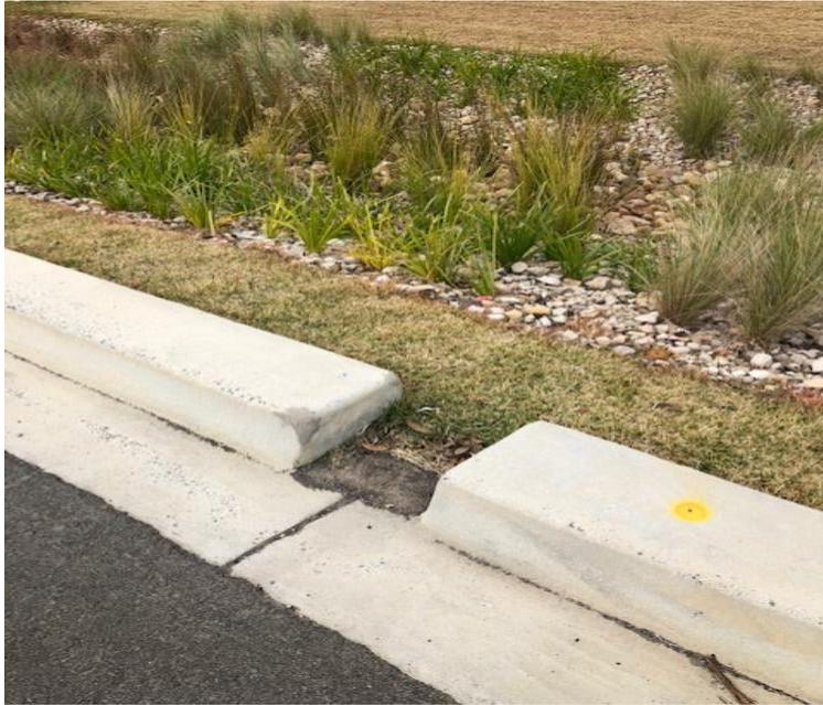
Road runoff is channelled into vegetated 'filter' strips for natural management of both volume and quality rather than transported into pits and pipes. *The Glenlee proposal lacks this treatment.*
