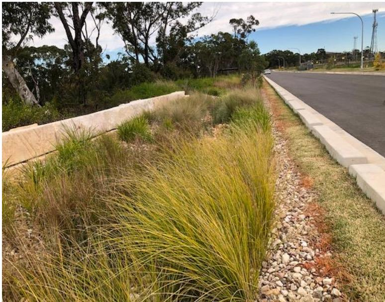
Before the subdivision meets the sensitive River riparian zone, an infiltration channel of pebbles and a rain garden is in place. It is effectively a buffer zone. *The Glenlee proposal does not provide such protection to the sensitive zones adjacent.*
